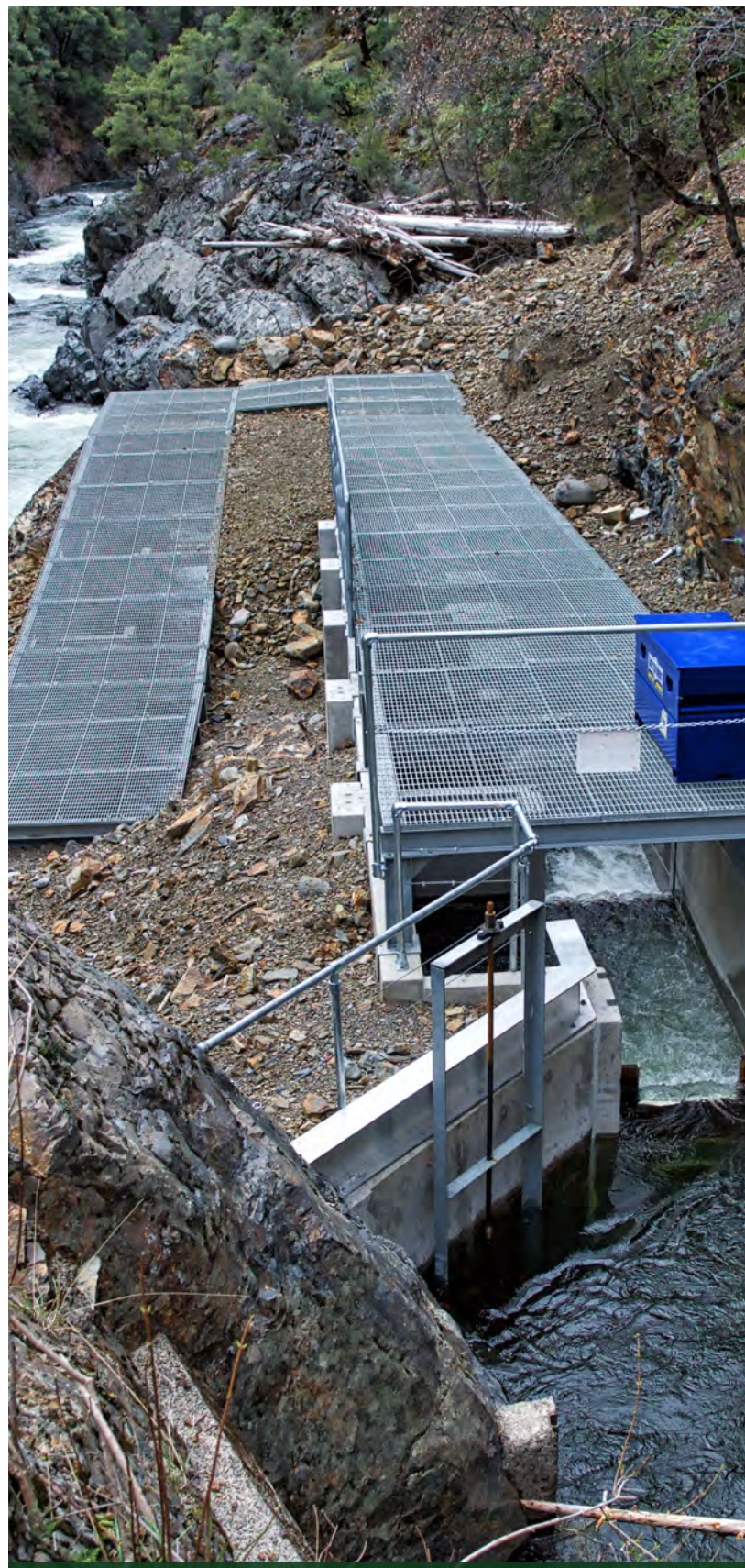
Lower Deer Creek Falls Fish Passage Improvement Project, Tehama County
